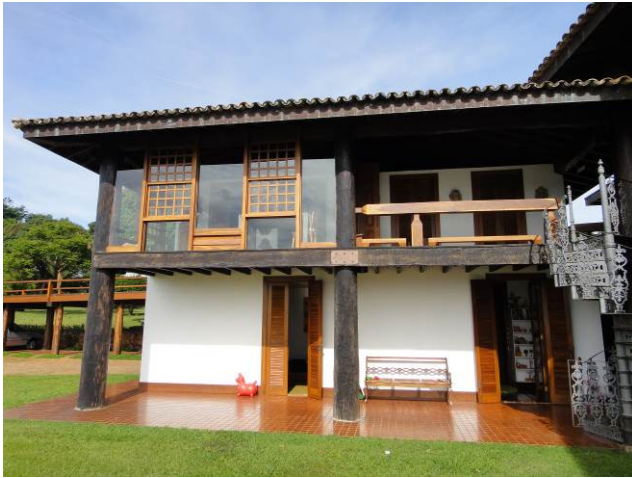
Figure 18 – Details of the walls and window wooden frames.
