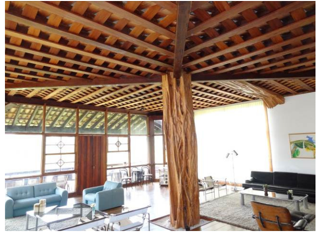
Figure 4 – Internal view of the ceiling, the central “acariquara” column in the foreground, and vertical enclosures at the back.
