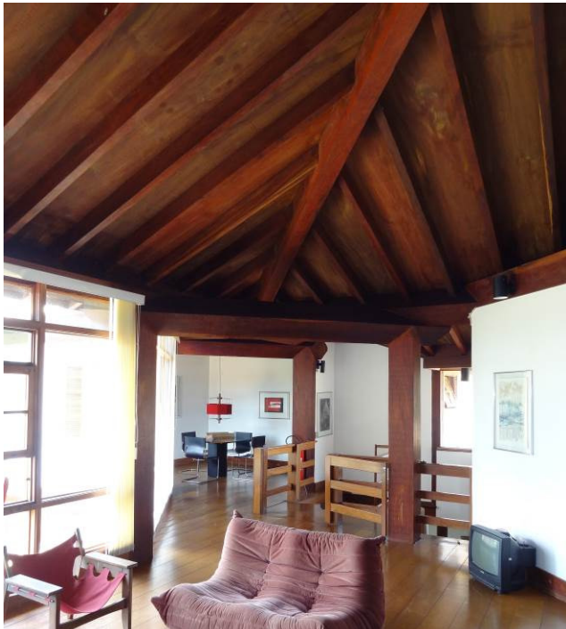
Figure 3 – Ceiling view at the junction of two slopes.
