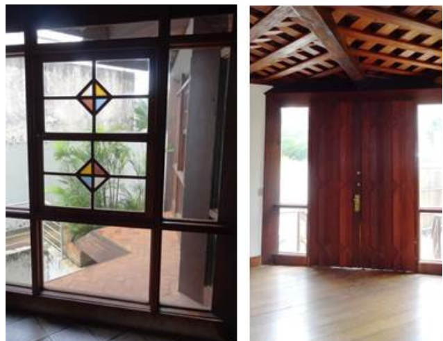
Figure 5 – Panels, window and door frames.
