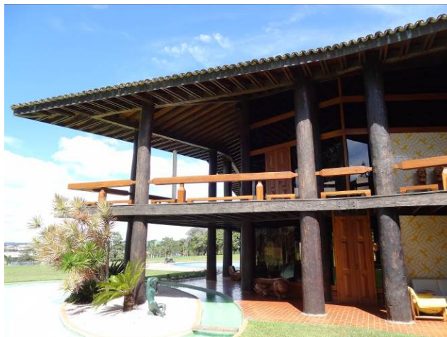
Figure 16 – Verandas and internal spaces enclosures.
