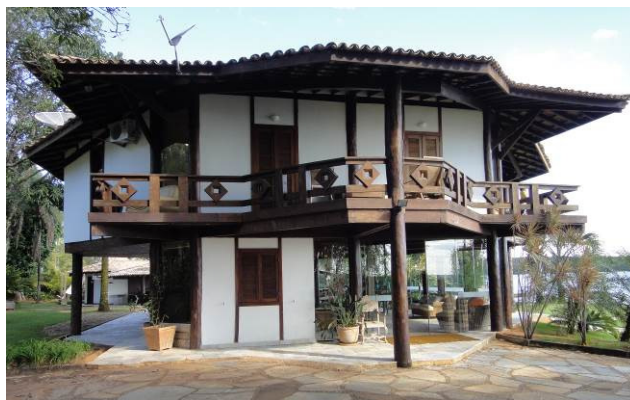
Figure 10 – Vertical seals and prolonged eaves
