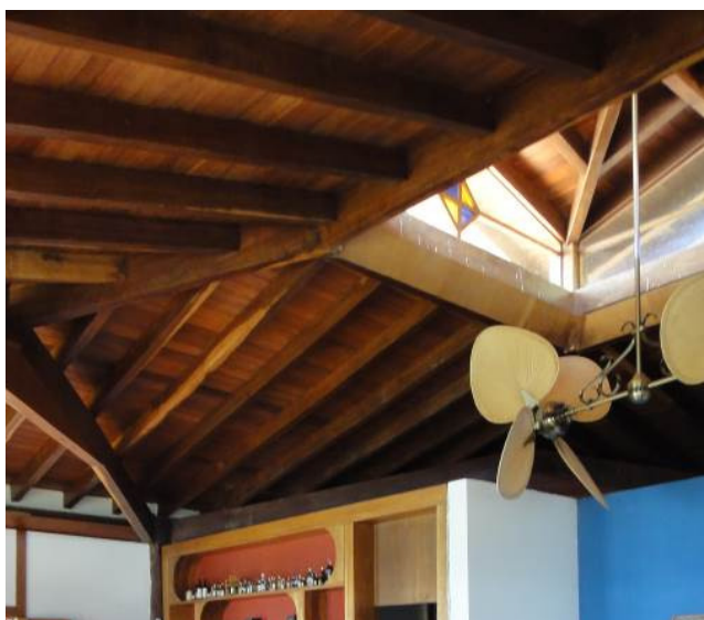
Figure 9 – The skylight and roof structure.
