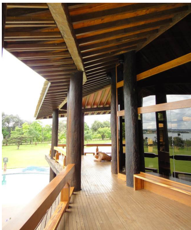
Figure 17 – Flooring and roof over the verandas.
