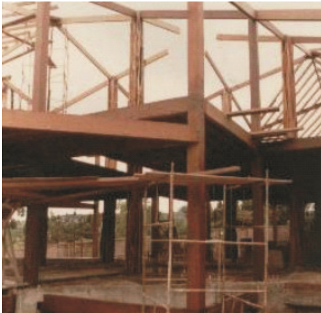
Figure 21 – Structure being built.
